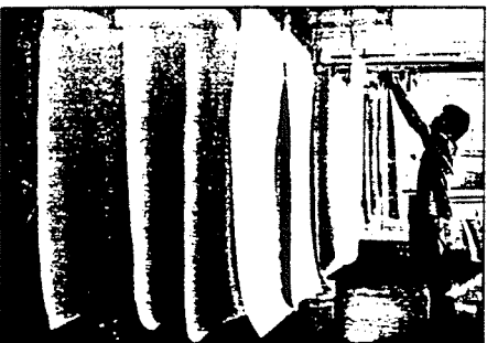
Hanging papers to dry in the drying loft.
